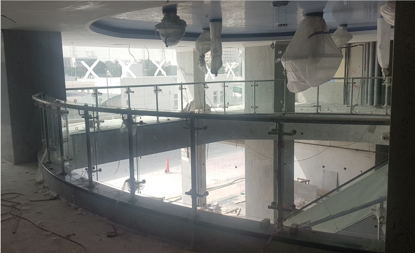
Rals Building Contracting, SS Handrail. Bin Shabib mall
